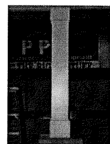
21) Clean surface of column with cleaner recommended by the paint manufacturer. Paint with 2 coats of acrylic latex paint.
