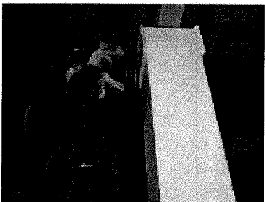
19) Option 2: Leave ¼" expansion room above cap, and pin-nail the cap to the column. Be sure pin-nails DO NOT reach the blocking inside!*
