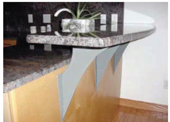
**As a general guideline countertops that are mounted to the wall or have no support other than the brackets are a heavy loading installation for brackets. In instances where the bracket is supporting the entire load of the countertop, gusset brackets must be used.**
